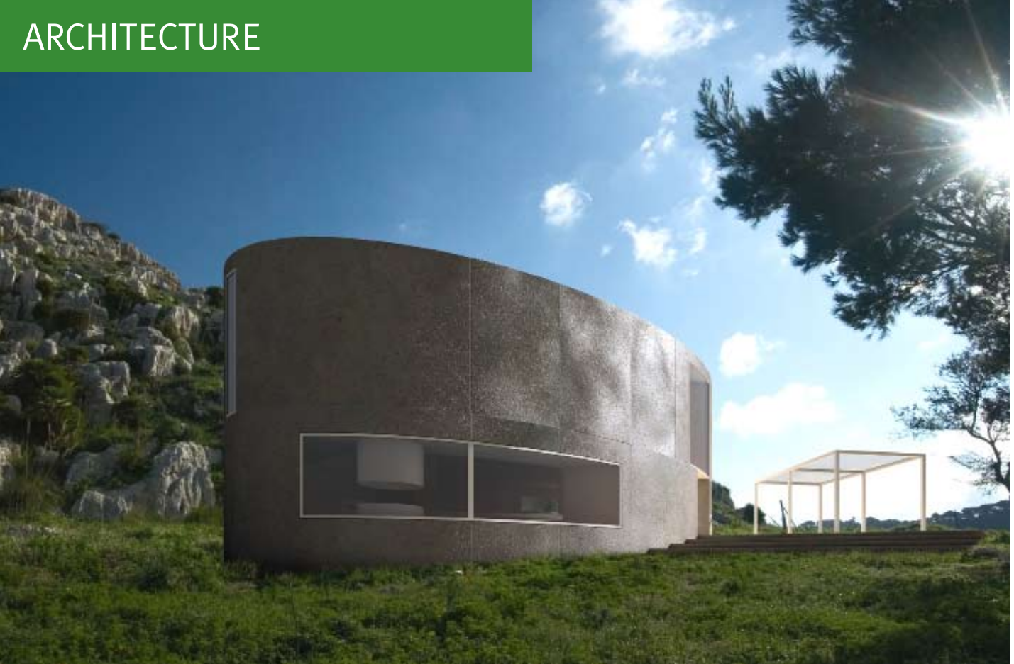
Monolithic castings of light-weight concrete forms the shell of the house that is climate and light sensitive
